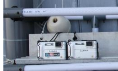
Fig. 1. Stereo Camera Installation
