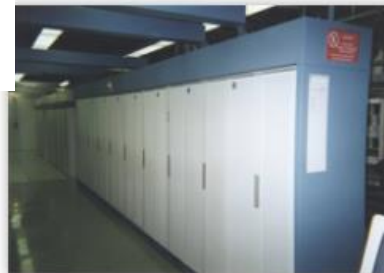
Large Telephone Switches
