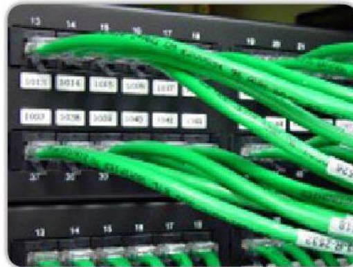
Front of Patch Panel
