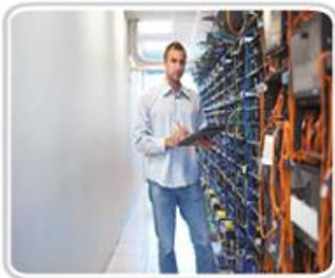
Installations must be inspected for damage.
