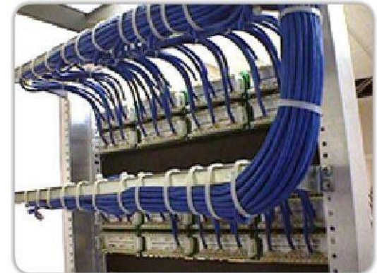
Rear of Patch Panel
