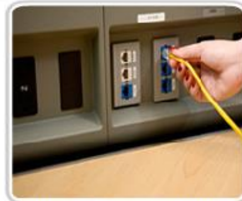
Cables must be connected correctly.
